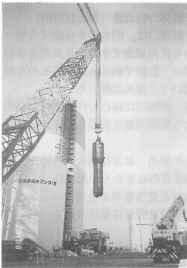
Photo 1 Carrying out of the old SG
